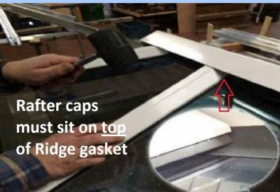
12. Tap rafter caps down on TOP of ridge cap gasket
