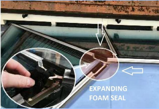
9. Push expanding foam strips in gaps on radius
