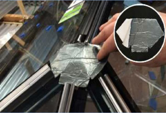
10. Apply adhesive cover to radius, covering foam seals
