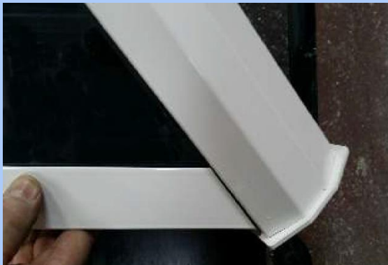
14. Position so glass end trim fits to edge of rafter
